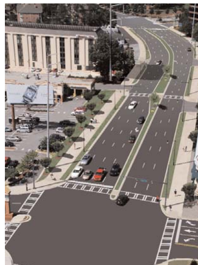
Wider sidewalks, raised/landscaped medians and dedicated left-turn lanes are just a few of the improvements recommended in the Piedmont Area Transportation Study.
